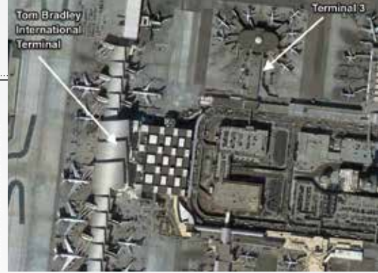
Terminal 3 and the Tom Bradley International Terminal at LAX. Conventional scanning surveys of the buildings would require several weeks of field work
